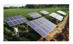
The solar pump using a solar energy system is an attractive technology with environmentally as well as socially for supplying the water in remote locations. So this is always an economically chosen technology. Generally, remote places mainly depend on diesel engines, manpower for supplying the water. These pumps replace the present pumps to
