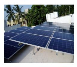
Solar rooftop are solar panels placed on top of roofs of commercial, institutional or residential buildings. They capture the light energy emitted by the sun and convert it into electrical energy. This setup is also known as *solar rooftop* photo-voltaic system. It produces a clean, Eco friendly form of energy, meaning that it's which does not produce any type of pollution or harmful gases.
